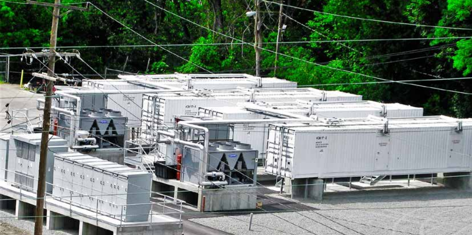
8 MW Li-ion battery grid storage system in New York State (Photo: AES Corporation)
